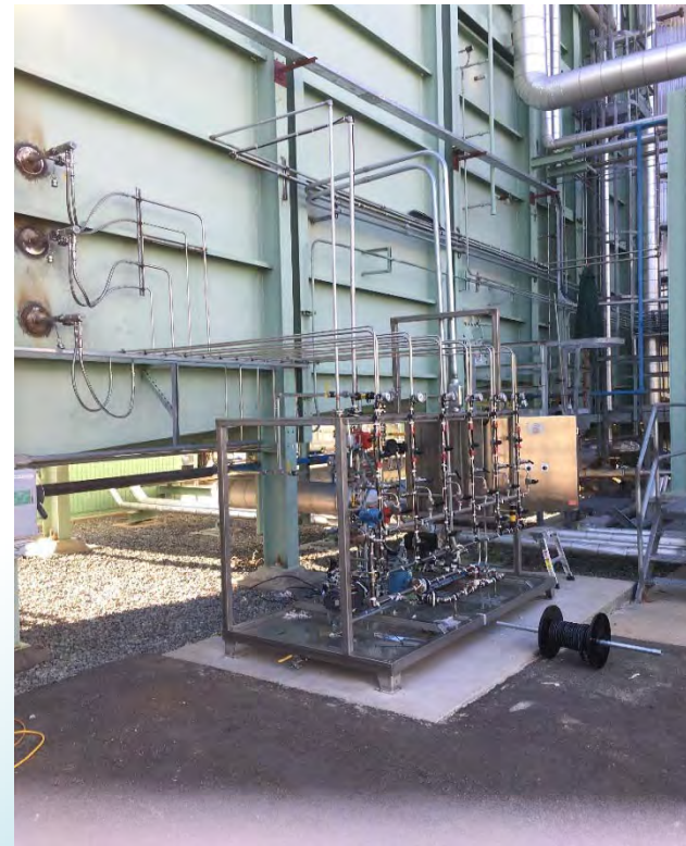
Liquid urea injection points
