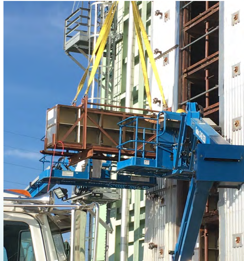
Use of module installation cart
