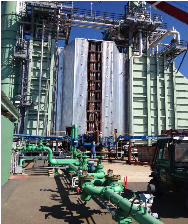
Four layers of catalyst
